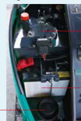
Hydraulic tank Battery
